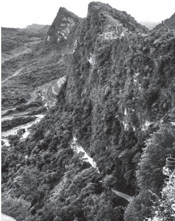
Fig. 4. Downstream face of the ridge in which the Yacambú dam is located. The downstream toe of the concrete-faced rockfill dam can be seen in the centre of the photograph
