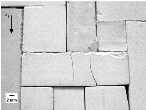
Fig. 14 Double cracking in the lengthy horizontal elements
