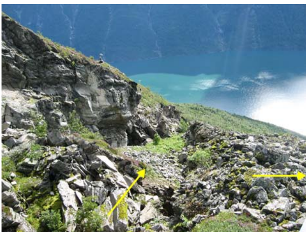
Fig. 19 Graben (block 6 in Fig. 6) looking towards ESE. The difference in the measured surface movement directions is indicated by arrows
