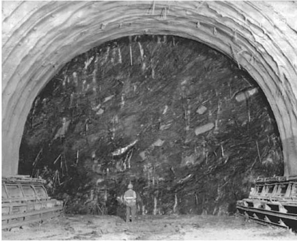
Fig. 17. Raticosa tunnel full face excavation (courtesy of Rocksoil, Milano)
