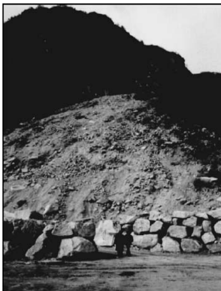
Fig. 2. Photograph of the Alps field test slope
