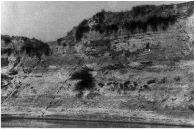
Fig. 6 Cliff section exposed at left bank of river Yamuna at Shergarh Ghat near Auraiya. The calcrete nodule bearing mottled silt and mottled silty fine sand units are cut by conjugate fractures. Note the tilt in the blocks away from the river channel (river flows on to the left-hand side of the photograph )
