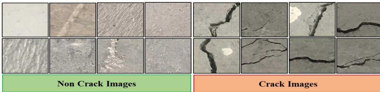
Fig. 11 Sample collection of crack and non-crack images
