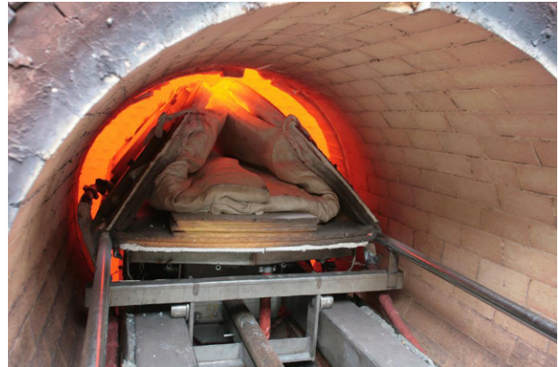
Fig. 8: Burner repair while maintaining hot blast system at operating temperature
