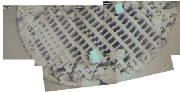
Fig. 4: Endoscopic Inspection for Assessment of Stove Internals
