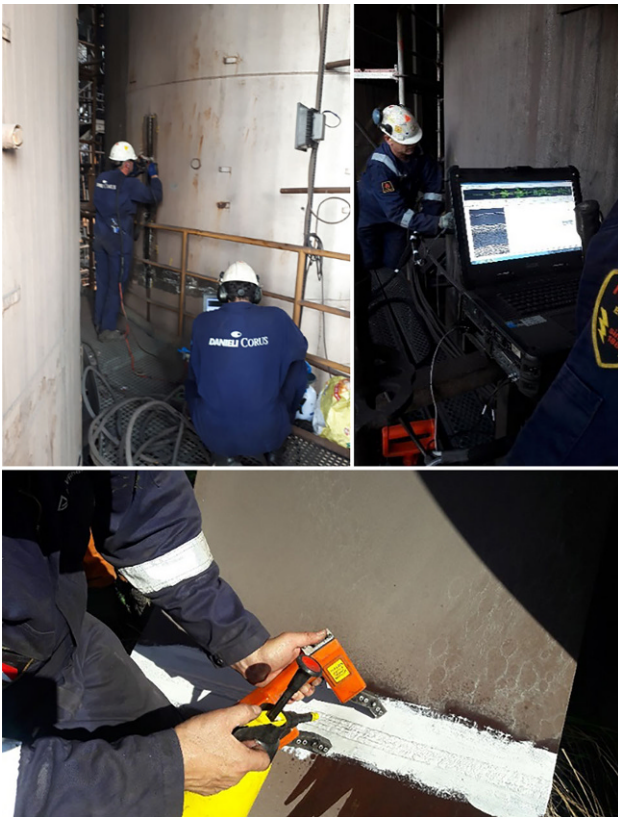
Fig. 3: Shell Condition Assessment, TOFD Measurement in Progress
