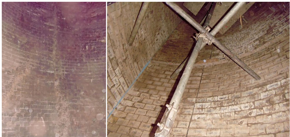
Fig. 9: Combustion Chamber before and after application of new refractory
