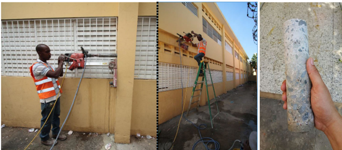
Fig. 15 Concrete core extraction
