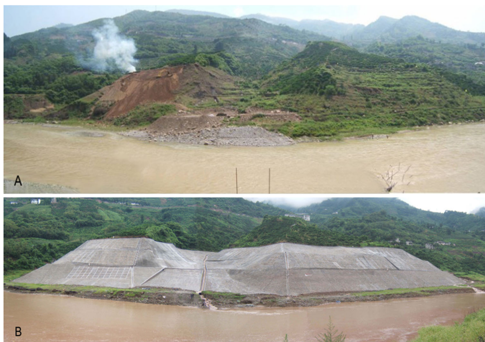
Fig. 11 Contrast photos of Jinle landslide before (a) and after (b) the implement of revetment measures
