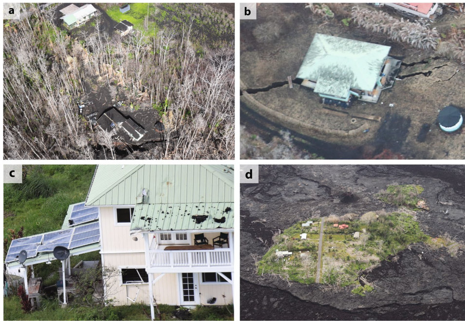
Fig. 14 Photographs taken from helicopters of a structures with white roofs covered in tephra, close to a fissure in the foreground; roofs of structures with tephra clean-up evident in the background. Vegetation damaged by gas and steam emitted from the fissures. Ground-surveys showed corrosion to structures from gas and steam impacts (taken 6 November 2018), b fissures that have opened underneath a
