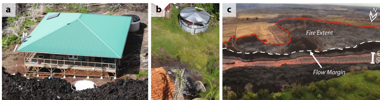
Fig. 13 Photographs taken during the lower East Rift Zone (LERZ) eruption of a a wooden dwelling not in contact with the lava flow categorised as DS1, with melting of plastic cladding caused by the thermal effects of the lava (taken 6 November 2018), b damage to a structure by fire classified as DS5 (foreground) and a metal water tank
