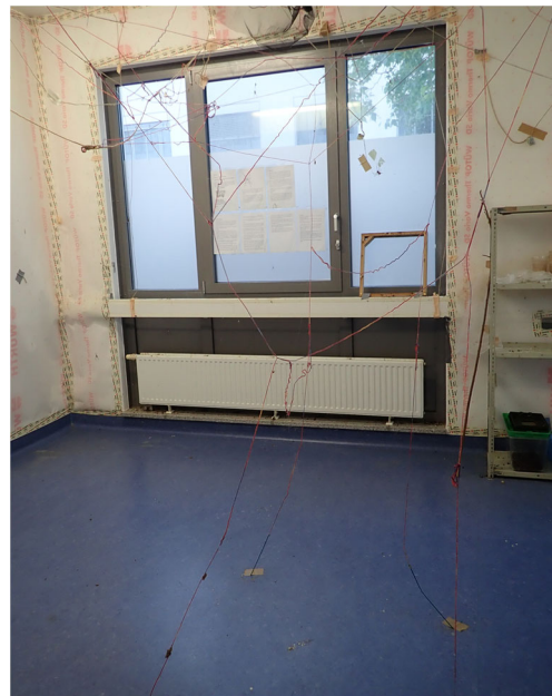
Fig. 11 Spider room at KRL with damp-proof interior, vapor retarding foil at the walls, and threads from floor to ceiling
