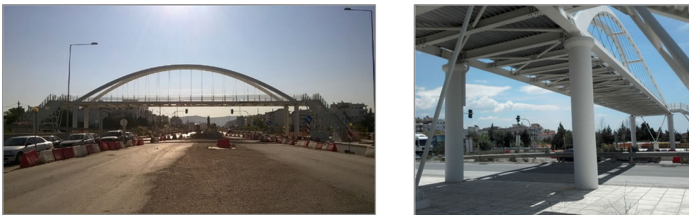
Fig. 8 The pedestrian highway overpass bridge
