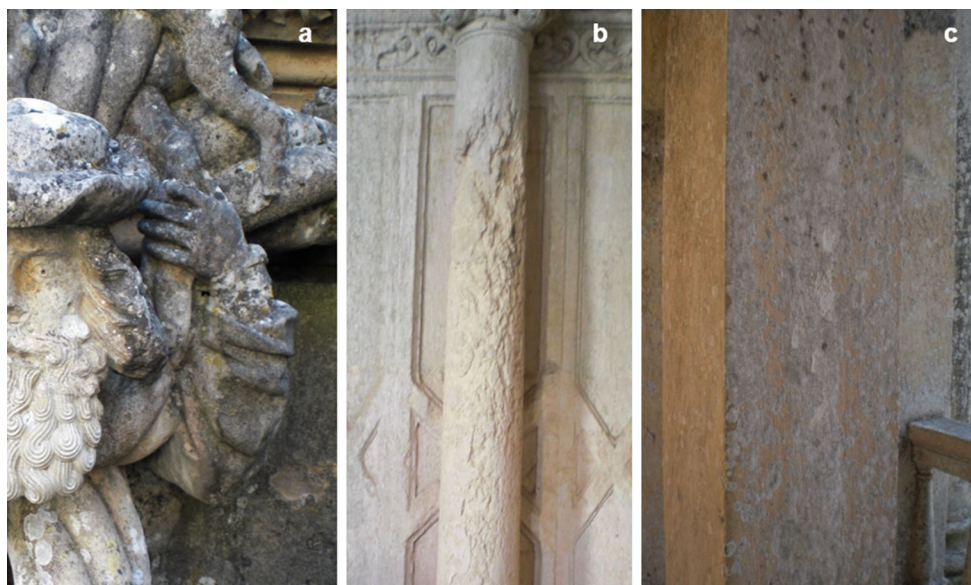
Fig. 1 Stone materials of Convent of Christ with evident alteration signs like coloured stains (a, b), structural degradation with fragments detachment (b) and biofilms formation (c) selected to evaluate their decay process
