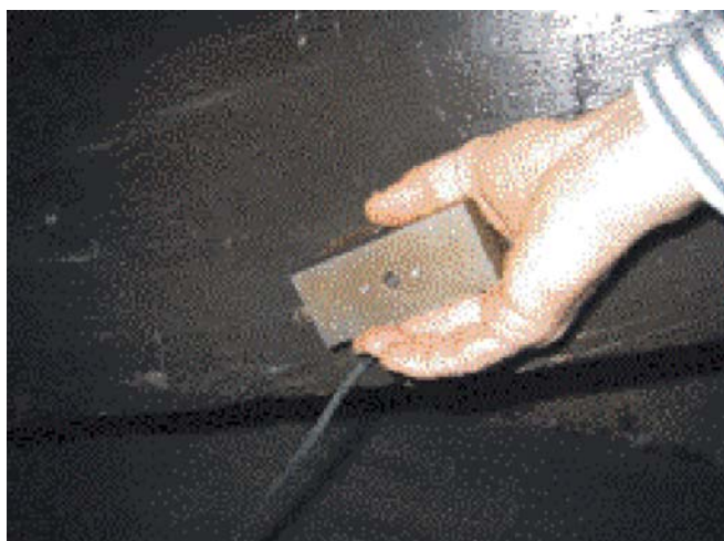
FIGURE 6 EM10 magnet and probehead during on-site measurements at “Torre delle Milizie” in Rome (Italy)
