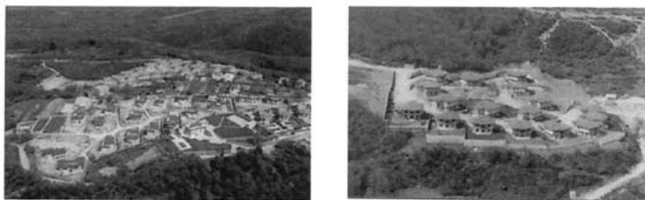
Figure 5. Aerial photographs for year 2000 showing the recent established residential sites within forest areas.
