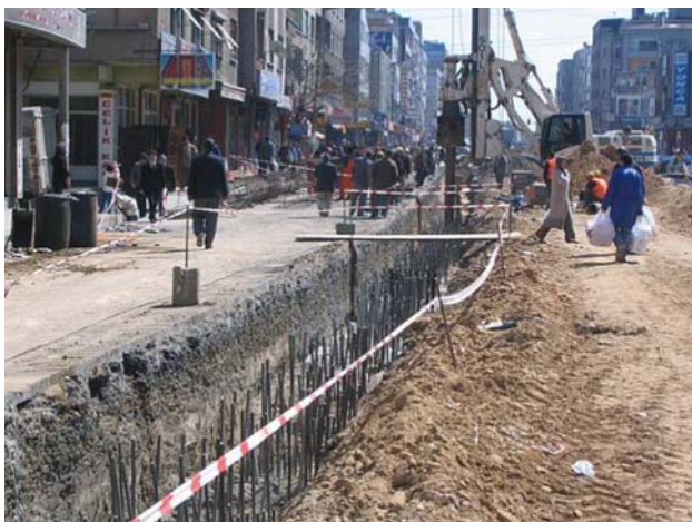
Fig. 9 Sultançiftliği–Edirnekapı tram construction and closed streets
