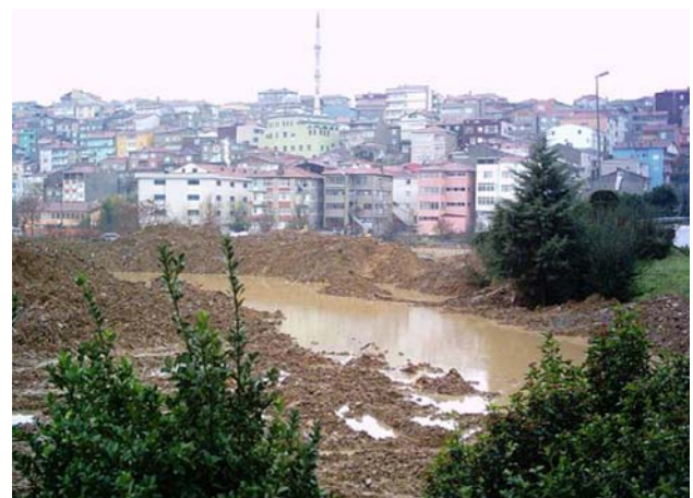
Fig. 7 Excavated material stocked for draining
