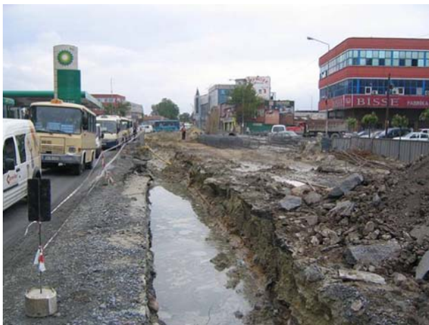
Fig. 8 Redirected traffic during tram construction
