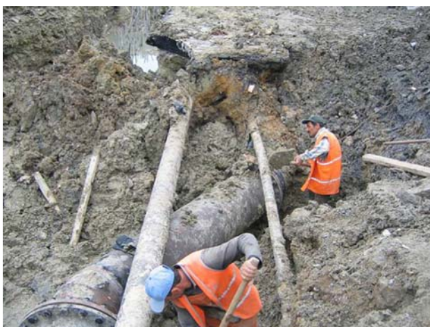
Fig. 12 Infrastructure transfers during metro excavations
