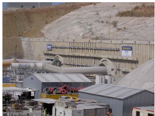
Fig. 8 Southern tunnel entrances at Abdalajís
