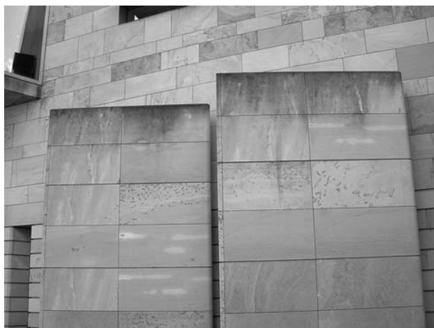
Fig. 1 The dark soiling developed along the upper edge of this stonework is largely biological in origin. Particulate soiling adheres to the sticky secretions of algae and other organisms which have colonised regularly wetted areas of sandstone
