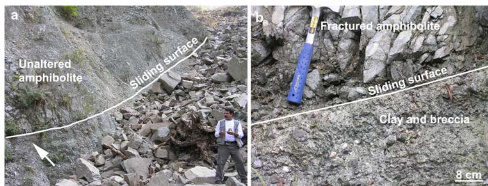
Fig. 11 Large-scale landslide at Location 16 along Narayangadh-Mugling Road and close view of slip surface and altered clay zone. Arrow in a shows the location of b
