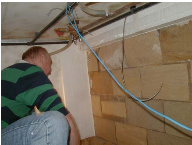
Fig. 3 Inspection of test wall in CERAM test chamber
