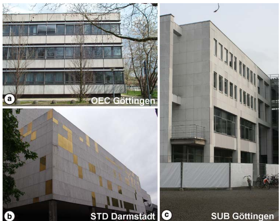
Fig. 2 Representative views of the facades from the a Oeconomicum, b State Theatre Darmstadt (STD) and c State University Library building (SUB). Critical panels of the STD are replaced by panels made from brass, while those from the SUB were replaced by fibre cement panels
