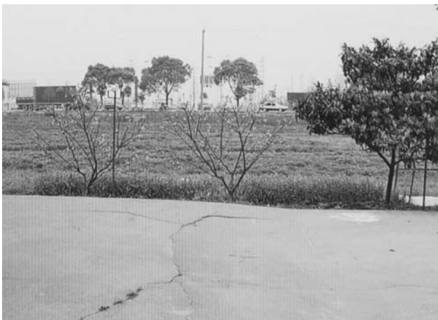
Fig. 12 An earth fissure induced by groundwater withdrawal
