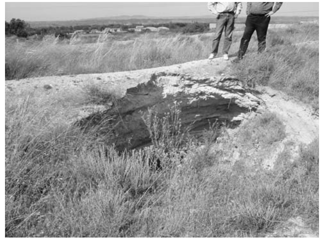
Fig. 4 Doline developed in an old section of the Canal Imperial de Aragón
