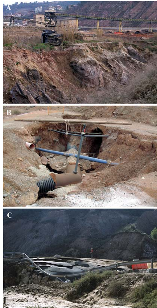
Fig. 11 Sinkholes induced by the March 1998 mine flood event in the vicinity of the Cardener River. a A composite collapse sinkhole generated in the Cardener River bed through which water sank into the mine galleries. b Collapse sinkhole affecting the brine collector at the confluence between the Riera Salada and the Cardener River. c Sinkhole affecting the old C1410a Road
