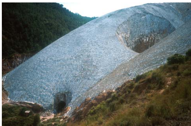
Fig. 5 The Old Slag Heap with the Sumider Gran, a collapse sinkhole 50 m across, generated in 1986. The origin of this doline is related to the upward sloping of the roof of a cave developed in the slag heap. The cave was largely excavated by sewage waters
