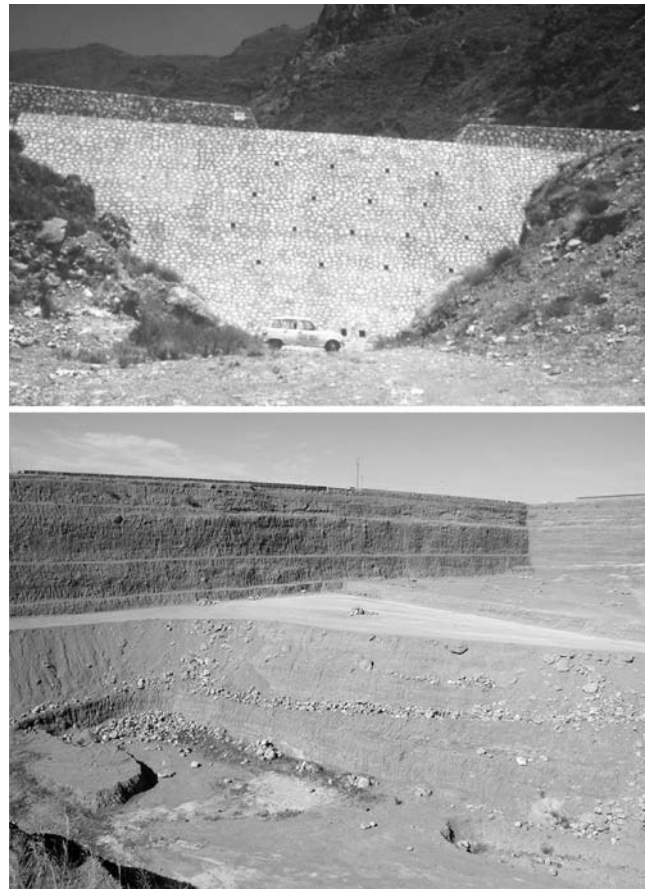
Fig. 2 A 13-m high masonry check dam in subbasin 32 (Águila subbasin), and view of one of the gravel pits in Carcáuz rambla
