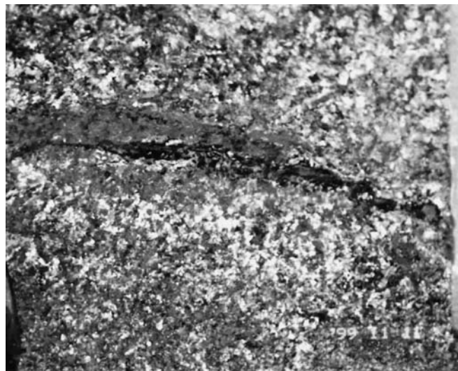
Fig. 3 Slip zone at trial trench TT1A
