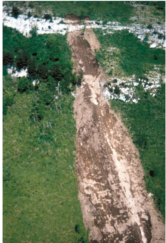
Fig. 8 Example of splash phenomenon downslope of a vertical limestone scarp in the Sarno area
