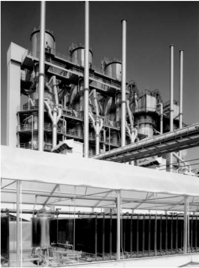
Fig. 2 Closed plate type photobioreactor fed with high CO 2 levels from a lime production plant in central Germany
