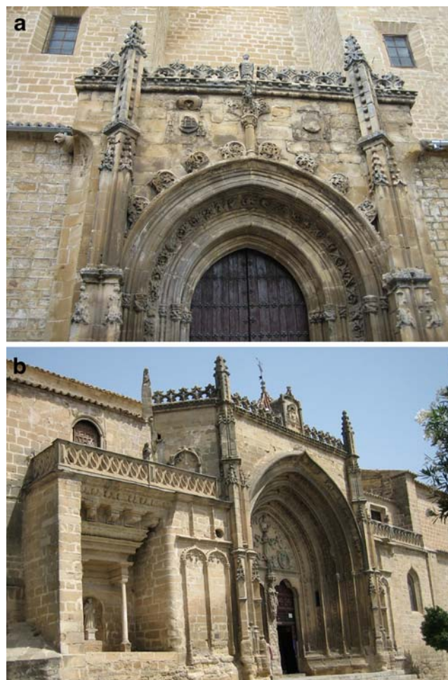
Fig. 1 Southern façades of San Isidoro (a) and San Pablo (b) churches in Úbeda (Spain)
