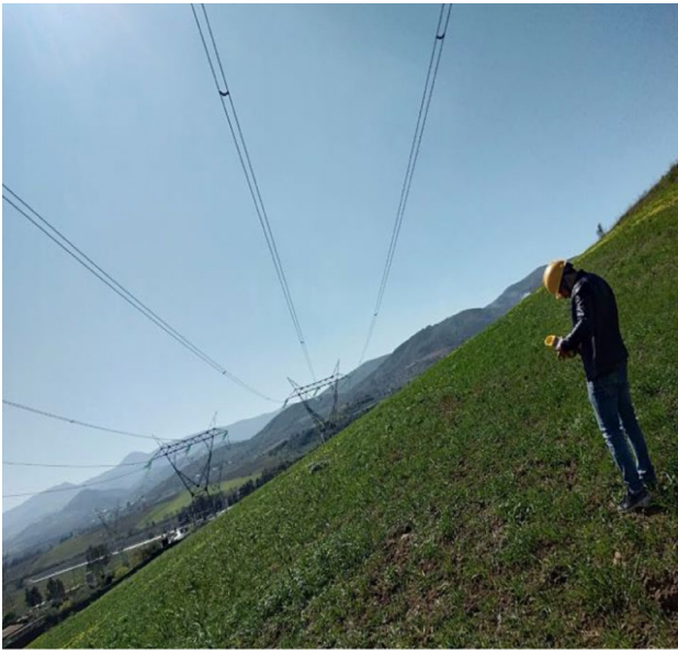
Fig. 7 Height measurement between ground and conductor
