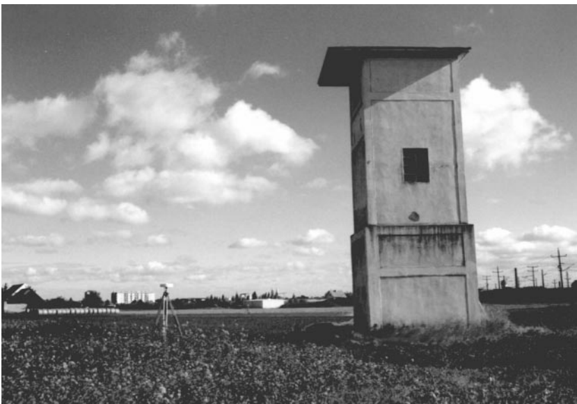
Fig. 6. The rover station beside the concrete building
