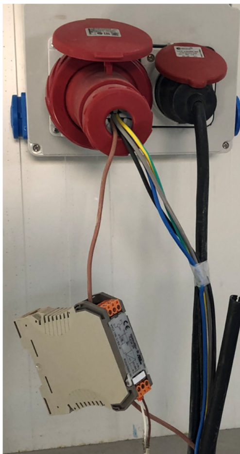
Fig. 11 Current sensor integration [18] (Copyrights reserved)
