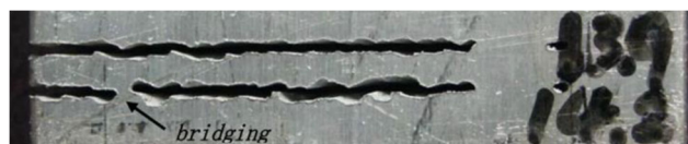
Fig. 2 Bridge generated in separation process
