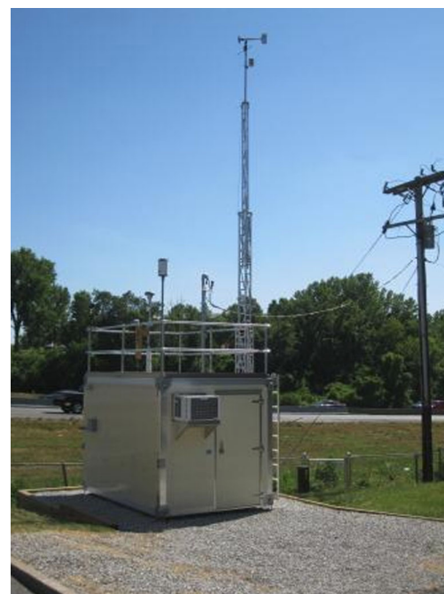
Fig. 2 Air quality monitoring station
