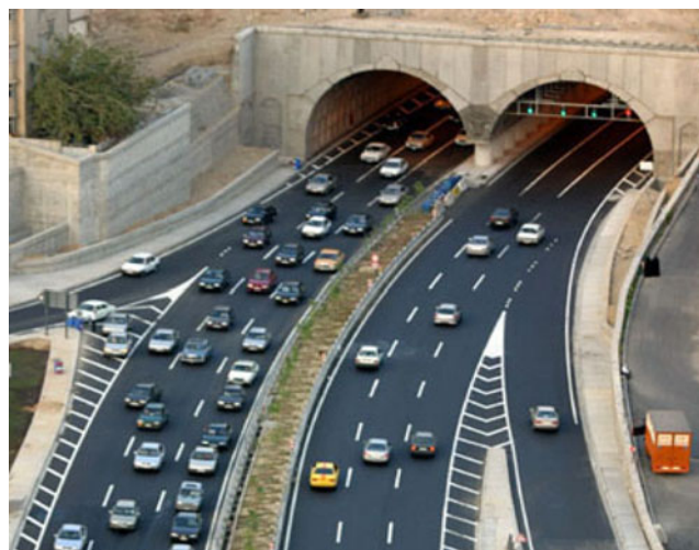
Fig. 1 Picture of Resalat tunnel
