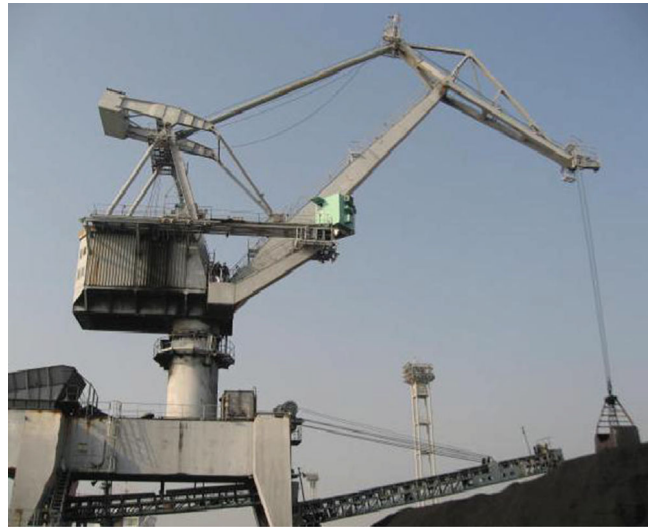
(a) General view of level luffing crane [3]
