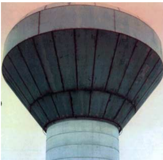
Fig. 18 Photograph of a typical elevated conical tank
