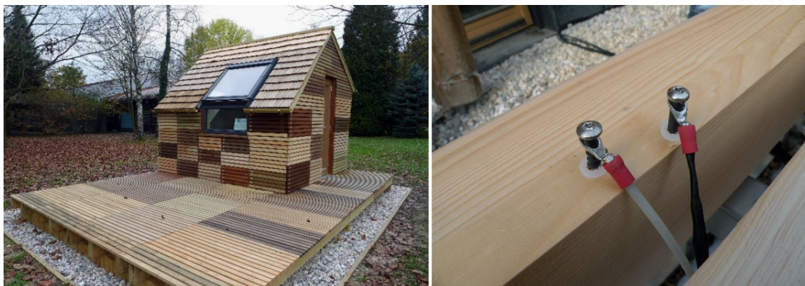
Fig. 1 Façade and decking of the wooden model house unit (left). Resistance sensors for MC measurements (right)
