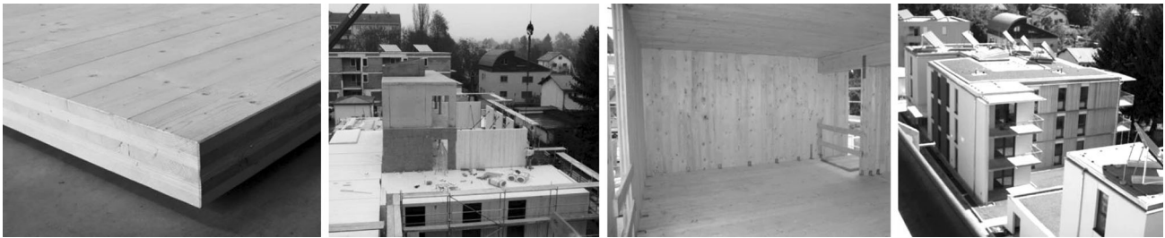
Fig. 1 (Left) five-layer CLT element; (middle to right) impressions from project Wittenbauerstraße/Graz/Austria: two three-storey residential buildings
