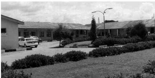
Figure 1. Front view of the Accident and Emergency Unit of the University of Ilorin Teaching Hospital, Ilorin, Nigeria.
