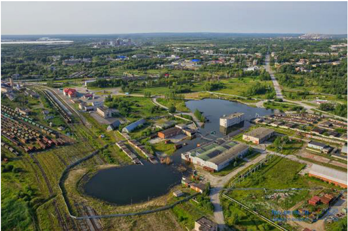
Figure 9 Technogenic lake at the location of sinkholes I and II in 2014
