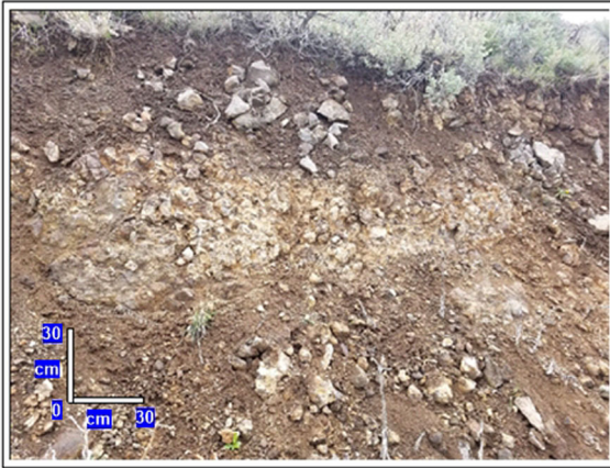
Figure 4 Road cut on Site 2 (the scale is approximate)
