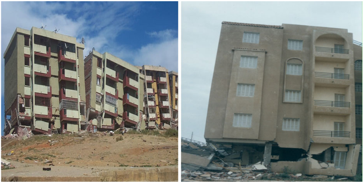
Figure 9 Typical damaged 4–5 story buildings in the Boumerdes area near the Boumerdes station (near source)
