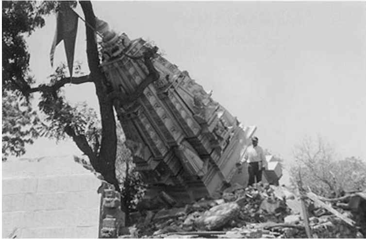
Figure 10 Overturned object at Adhoi (23.4°N, 70.5°E). (b/h) = 0.61.
