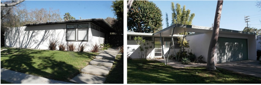
Fig. 1 Views of Mar Vista housing units: view of a standard unit (left), a unit with a large overhang where columns act as a unique additional element of the house (right). Photographs by the authors
