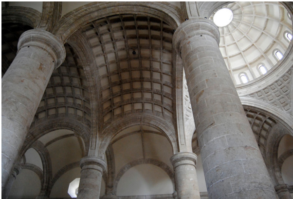
Fig. 13 Grid-crossing vaults of the San Ildefonso Cathedral, Mérida, Mexico
