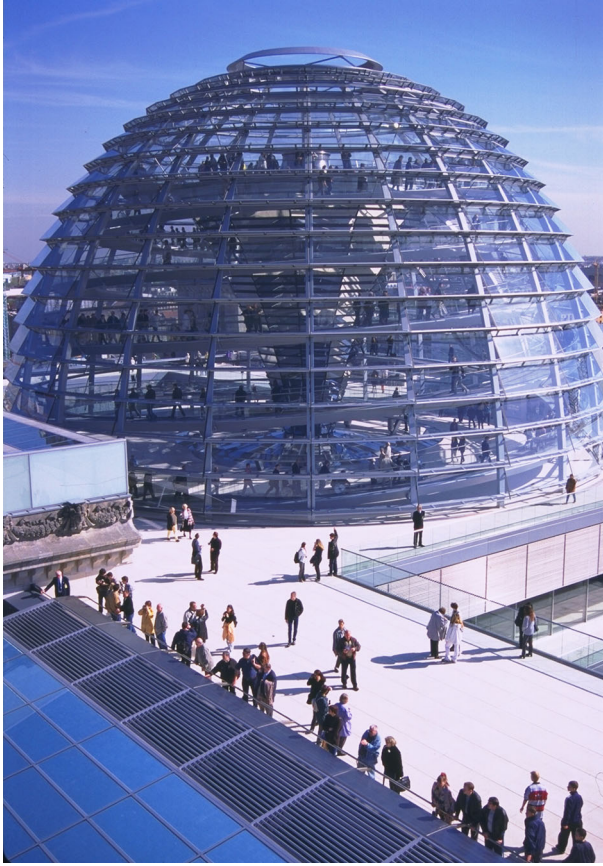
Fig. 9 The glass vault of the Reichstag divided in parallels. Courtesy of Foster + Partners
