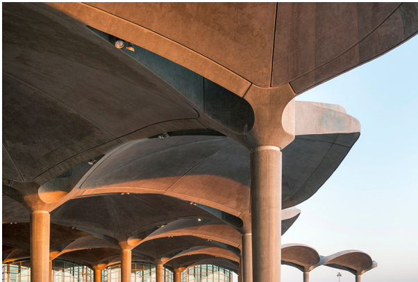
Fig. 19 The roof of Queen Alia International Airport
