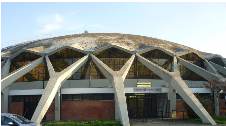
Fig. 2 Internally ribbed shell dome, Palazetto dello Sport, Rome, 1957–59 (Photo: Gabriel Tang)
