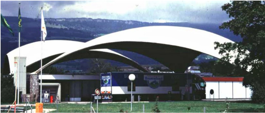
Fig. 8 The 31.6 m span shells for Deitingen Süd Petrol Station (1968) (Photo: John Chilton)
