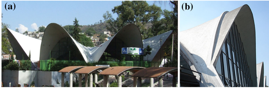
Fig. 3 a Los Manantiales Restaurant, Xochimilco, Mexico, 1958—Félix Candela, architectural design Joaquin and Fernando Alvarez; b stiffening rib, Bacardi Rum Factory, Cuautitlán (Photos: Marisela Mendoza)
