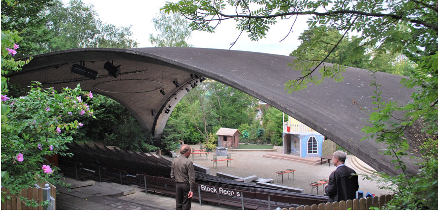
Fig. 9 The 42 m span shell for Grötzingen Open Air Theatre (1977) (Photo: John Chilton)
