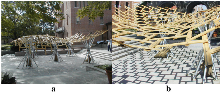
Fig. 2 Forest Park Pavilion: a view of the whole structure (Reproduced by kind permission of Shigeru Ban Architects. Source: http://www.shigerubanarchitects.com/works/2002_bamboo-roof/index.html ); b detail on the irregular disposition of element ends in a fan (Reproduced by kind permission of Cecil Balmond. Source: http://balmondstudio.tumblr.com/image/99042621238 )
