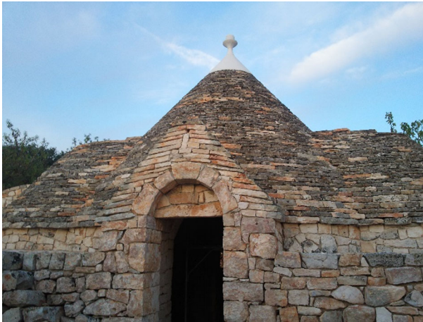
Fig. 12 Roof cladding made of chiancarelle to facilitate the water drainage
