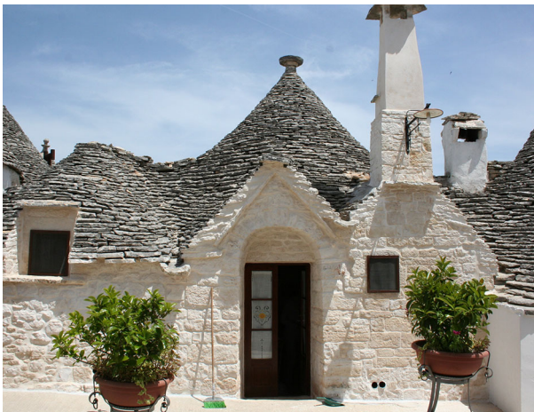
Fig. 1 Photo of a typical trullo located in the historical centre of Alberobello (Apulia)
