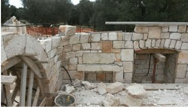
Fig. 9 Corner blocks to guide the construction of the candela
