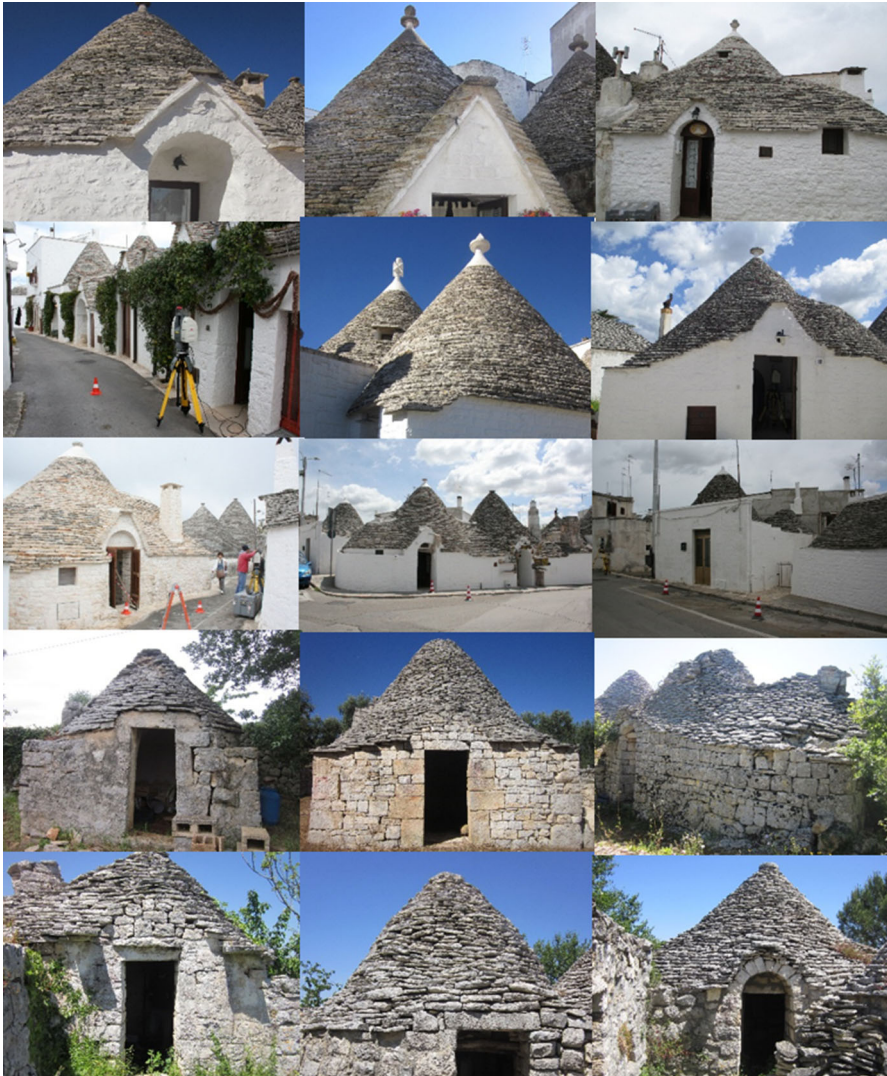
Fig. 2 An overview of the case studies (one of two) considered in the Apuliabase Project. The case studies belong to a wide range in terms of preservation conditions; both well-preserved and crumbling trulli were considered within the city centre (Alberobello) and its countryside
