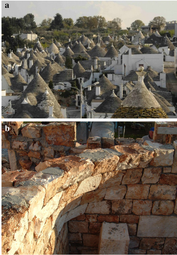
Fig. 5 Trulli are vernacular constructions mainly located in Valle d'Itria, an area between the cities of Bari, Taranto and Brindisi a an overview of Alberobello, the city with highest concentration of trulli; b a trullo during its construction
